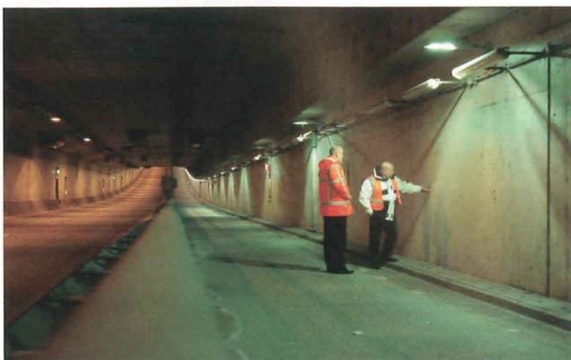
3600 Watt replaced by 160W in total
